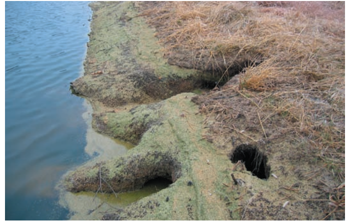
Figure 2. This neglected lagoon shows animal damage, poor grass care.
