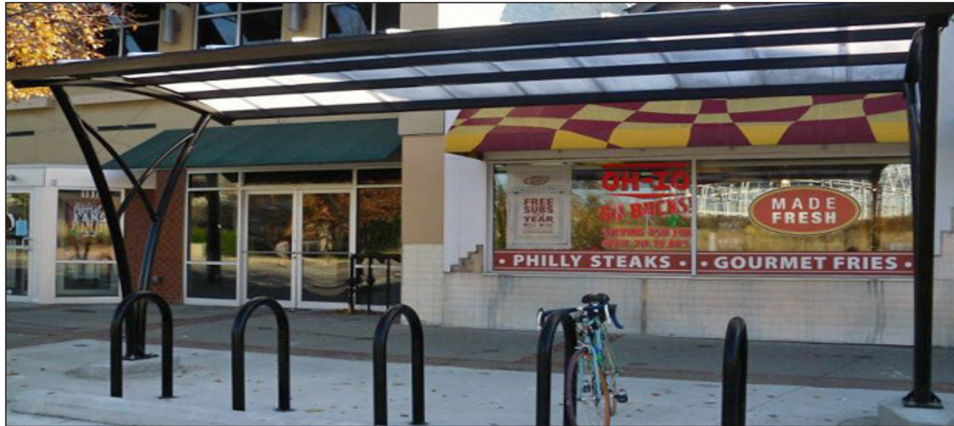
These “Inverted U” racks support a bicycle in two locations rather than just the wheel and are intuitive for users. Although the tubing is round, its thickness provides good strength.
