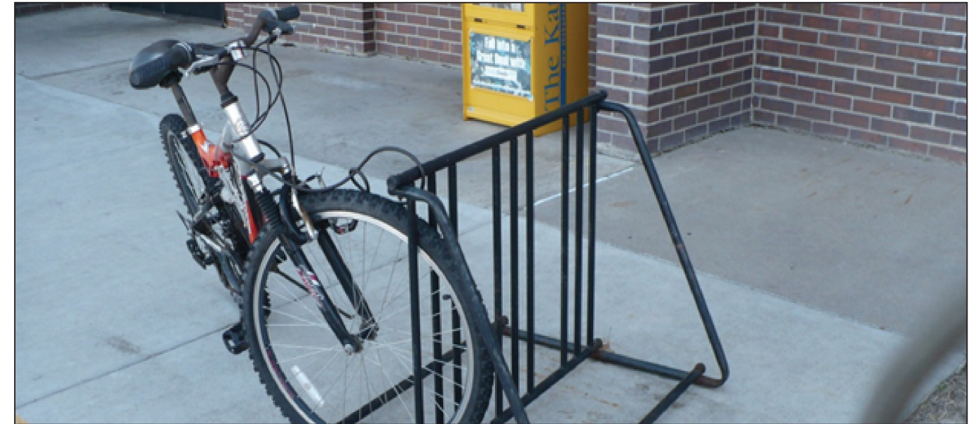
By supporting a bicycle at only one location, this grid rack puts pressure on the rim of a bicycle. Due to the spacing of the rack, the handlebars of different bicycles are likely to tangle.
